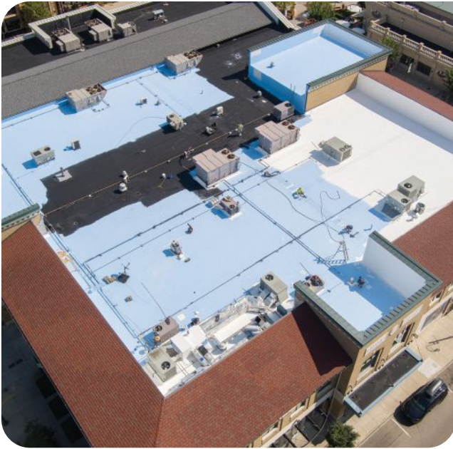
Liquid-applied membranes can significantly extend roof lifespans by up to three decades or more.
