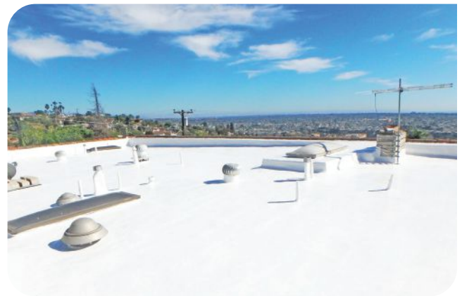
Along with lowering temperatures, cool roof systems also slow material wear, cut energy costs, and improve comfort for building occupants.
