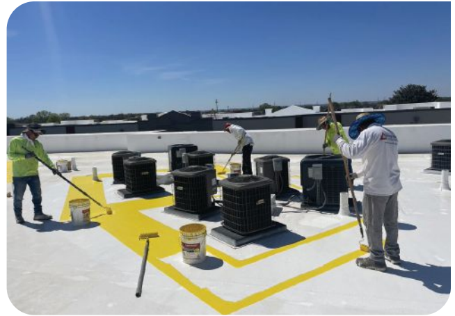
At the end of a warranty term, most sustainable roof coating systems may be reinstalled without requiring significant changes to the existing substrate.
